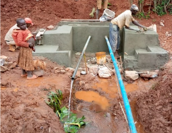
Figure 5: Unfinished spring catchment area in Burundi
